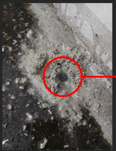
Presence of water beneath roof slab
