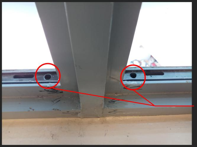
**Drilling additional** weep-hole to drain off water.
